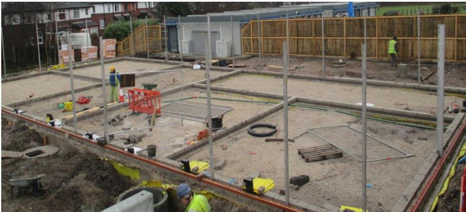
As you can see the new classroom build is progressing very well. It is now quite easy to see the footprint of the new extension and classrooms. The foundations are now in place and gravel has been put in and 'wackered', which is a process used to compress materials by using a machine called a compactor or 'wacker plate'! This is done to seal the ground in preparation for the pot and beam floor to be laid.
