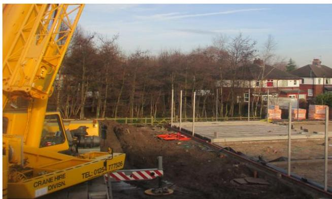
Above shows the start of the pot and beam floor being laid, this takes a 50 tonne crane to lift and position the flooring into place. Fun fact: 50 tonnes is about the weight of 6 African bull elephants!!!
